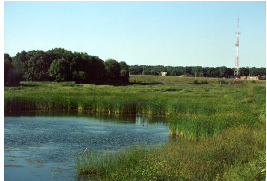
Douglas Road Landfill Leachate Treatment Wetland IN (courtesy Jim Bays Jacobs Engineering)
