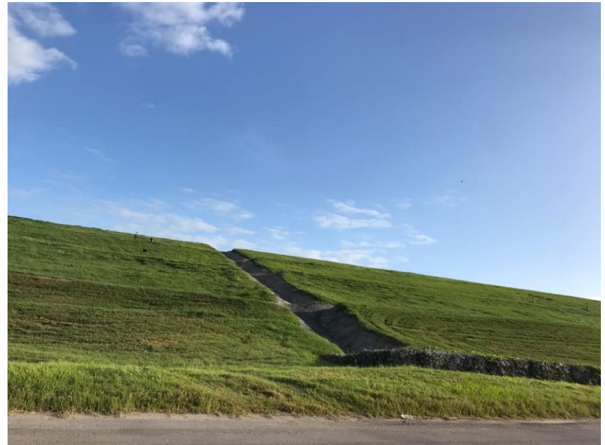
Southeast Hillsborough County Landfill in Lithia, FL
